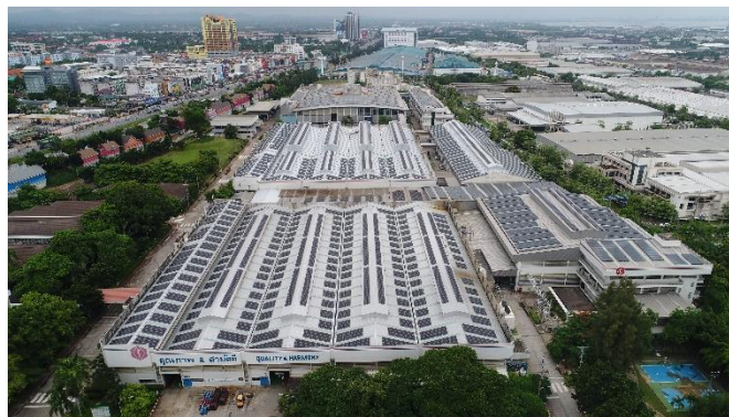
Siam Compressor Industry Co., Ltd
